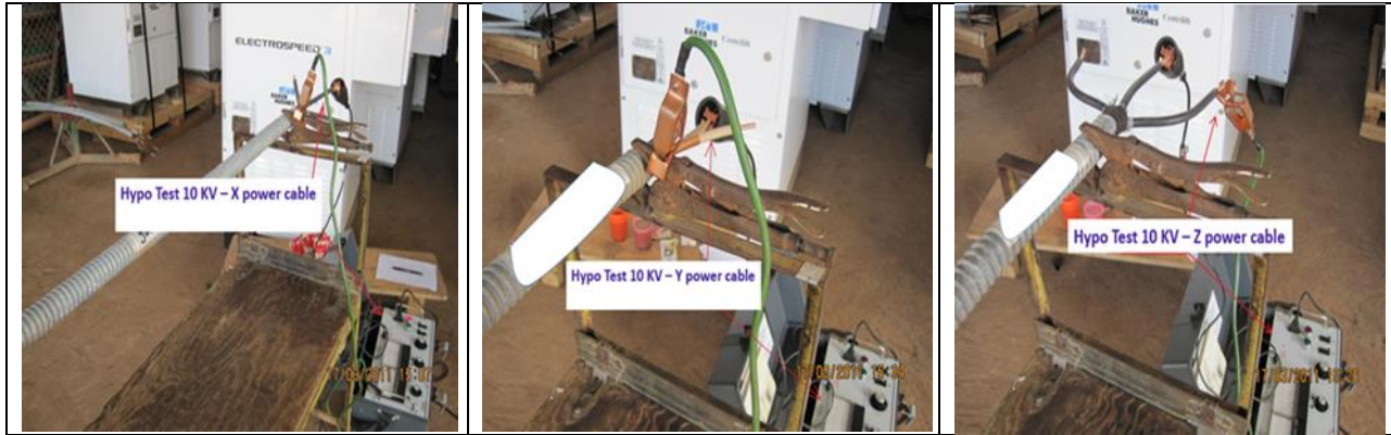
FIGURE 6: Hypo test 10 kV of X, Y, Z power cable results
