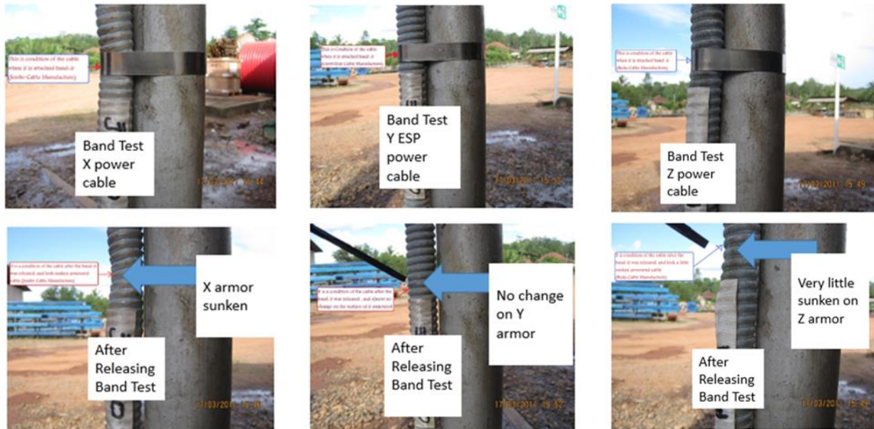
FIGURE 5: Band test result of X, Y, Z ESP power cable
