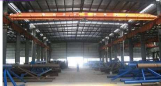
Figure 2 Overhead crane hoist to lift the cut plate to the assembly line.
