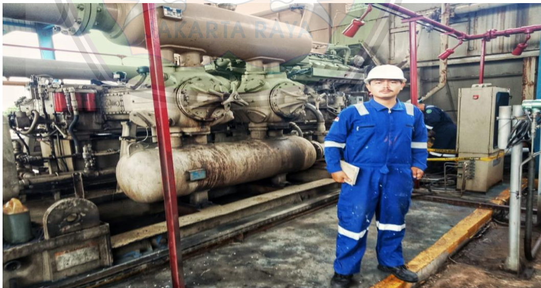
Gambar 1.1. Mesin Gas Engine
