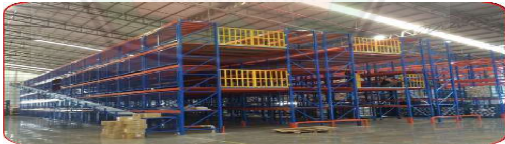
Gambar 1.1 Heavy Duty Pallet Racking
