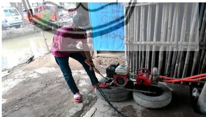
Gambar 1.3 : Proses Pengoperasian engine spray
